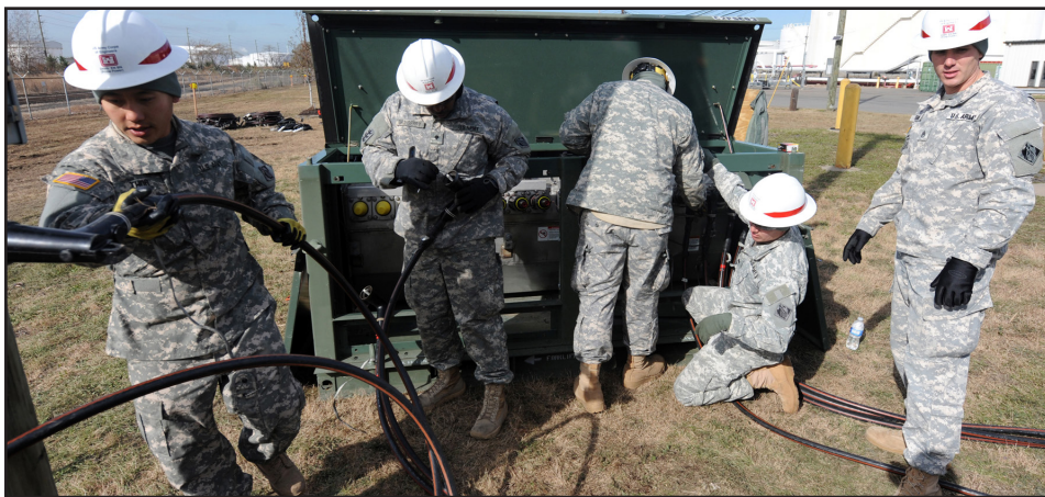
Soldiers with C Company, 249th Engineer Battalion (Prime Power), based out of Fort Belvoir, Virginia, install electrical generator equipment Nov. 6, 2012, at a Carteret, N.J. fuel depot that lost power during Hurricane Sandy. This work was critical to relieving gas shortages experienced by recovering communities in the immediate days following the storm. (Department of Defense photo by EJ Hersom)
