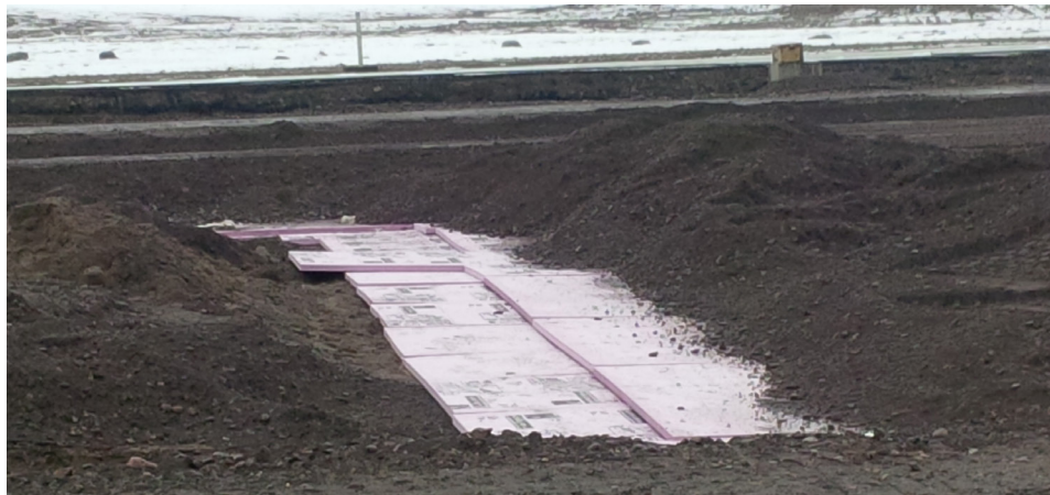
U.S. Army Engineer Research and Development Center researchers successfully attempted a repaving design that incorporated buried extruded polystyrene (foam insulation boards) to prevent permafrost thaw at the most critical locations on the Thule Air Base runway in Northwest Greenland. (Photo by Kevin Bjella)
